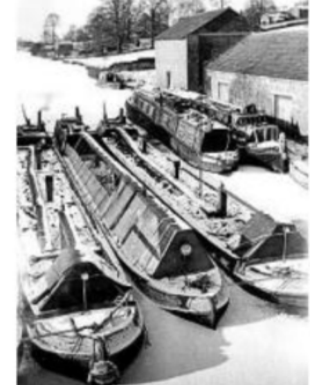
Braunston Bottom Lock during the terrible winter of 1962/3 when the canal froze for three months, helping to kill off what little trade remained on the canals. Three loaded Willow Wren boats are moored below the lock. Michael Street's pair of hotel boats – converted former working narrowboats – are moored against the quay. The buildings seen are the workshops of Willow Wren. PHOTO: PAT STREET
