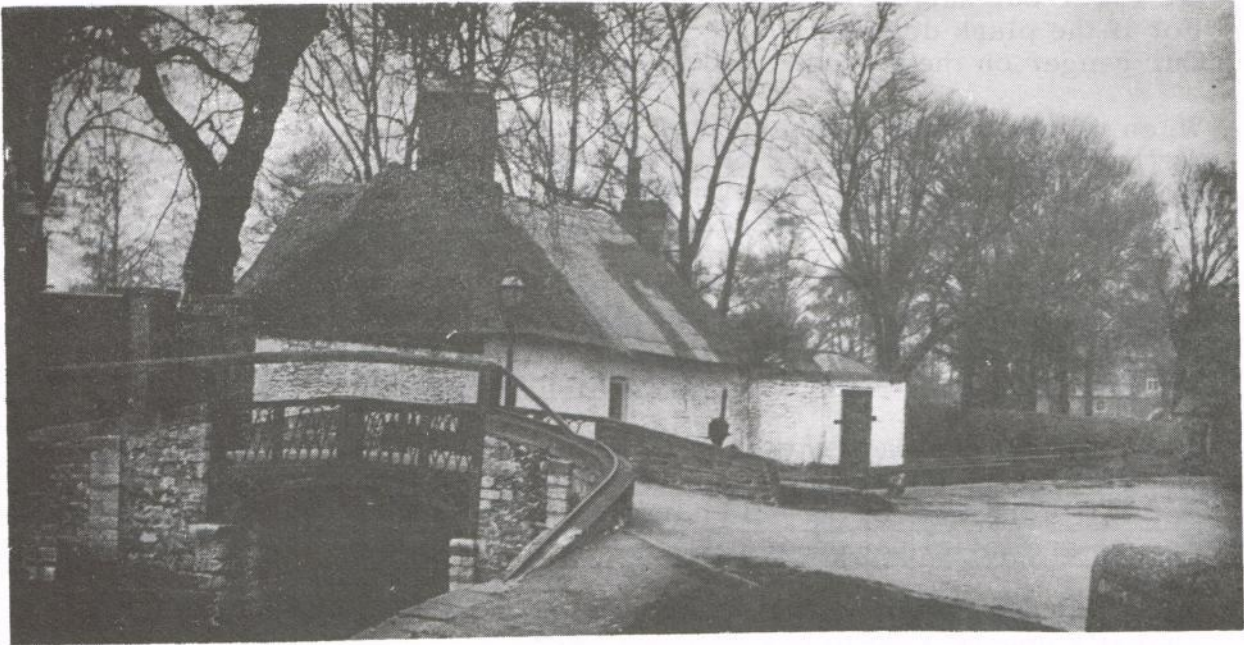
The Lock Keepers Cottage, near Cardiff Castle, on the Glamorgan Canal. Photograph: Leonard Raven (1939).
